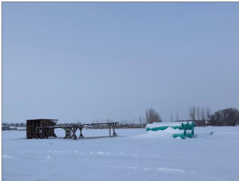
Photo 4 – Building materials storage on the south portion of the Site.
